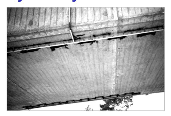
A chain of overlapping 300 mm long strain gauges were placed along each corner
