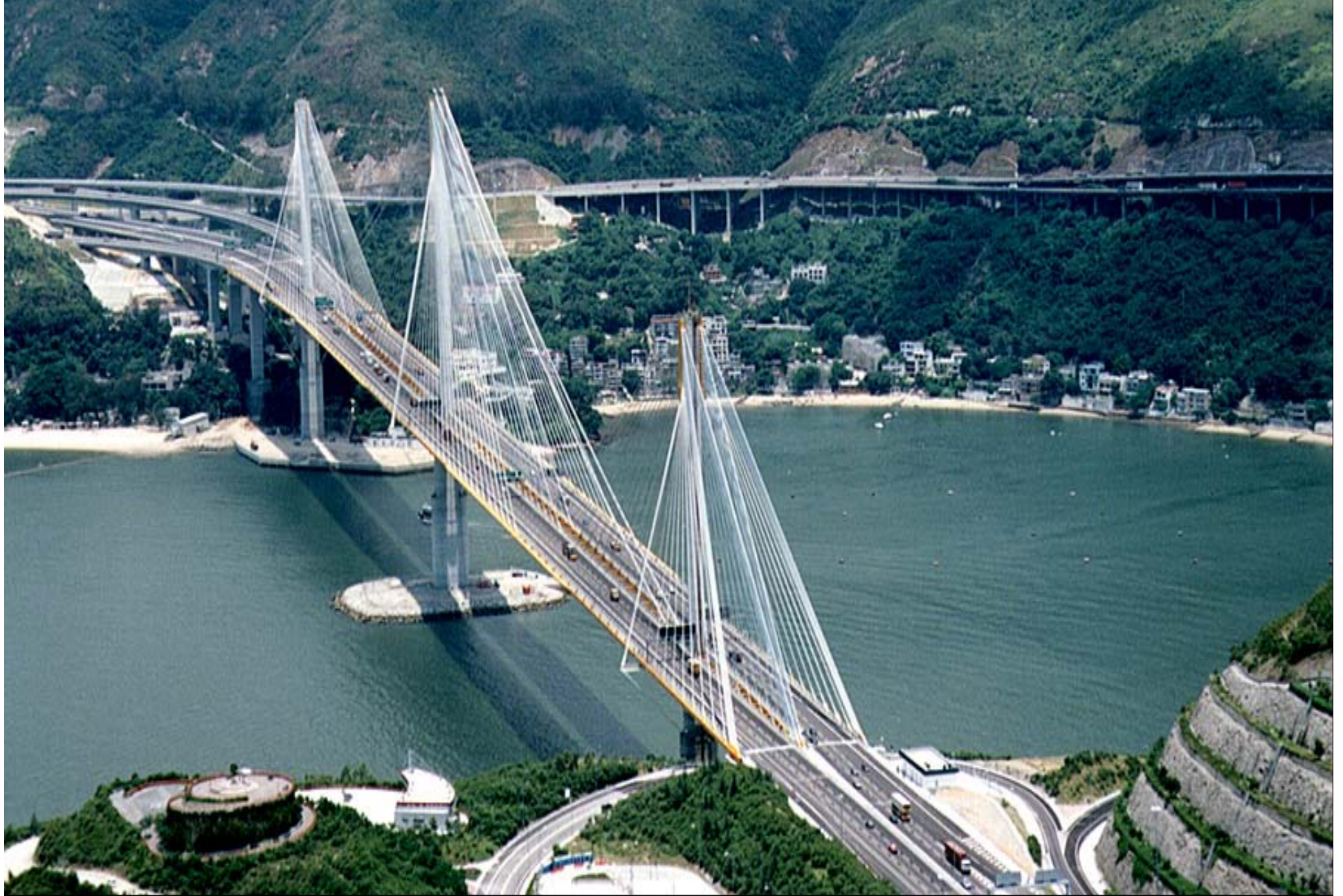
Ting Kau Bridge
