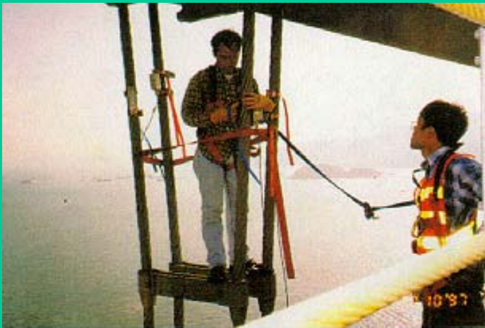
Field Measurement Works on Tsing Ma Bridge
