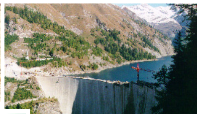
SOFO® System Dam Monitoring
