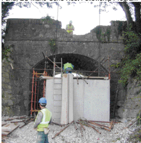
Greenfield's Bridge, Co. Cork, Ireland – high level load testing
