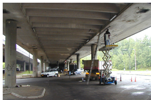
▲ Installation of 5 m long optical fibre sensor (DEF) for deformations
