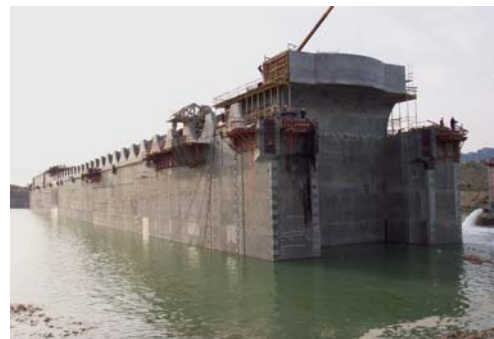
▲ Figure 1: The caisson during the controlled flooding of the basin
