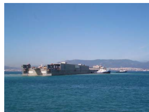
▲ Figure 2: The caisson during the transport to Monaco
