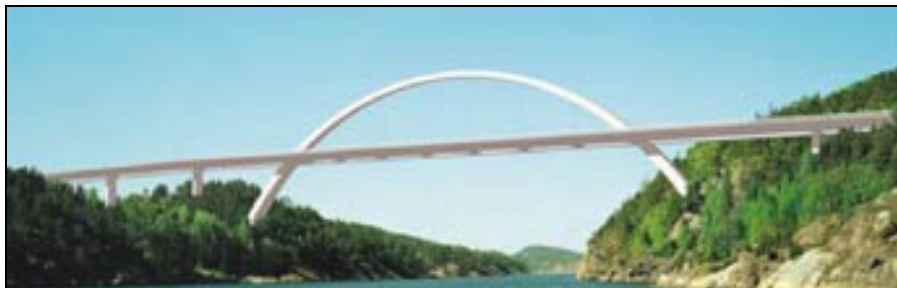
Fig. A.2.1. An artist's impression of the New Svinesund Bridge joining Sweden and Norway. The main span is a single arch with a bridge deck on either side of the arch.
