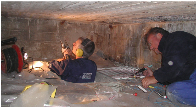
Fig. A.1.6. Installation of sensors in cell over parking lot (the third person is behind the camera).
