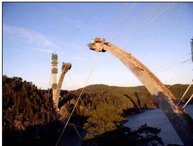
Fig. A2.2. Photograph of the arch under construction.
