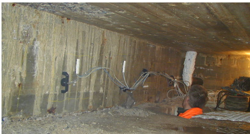
Fig. A.1.7. The cell over the railway after the sensor installation.
