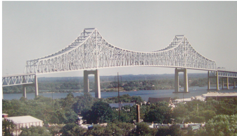
Commodore Barry Bridge Through-Truss Structure
