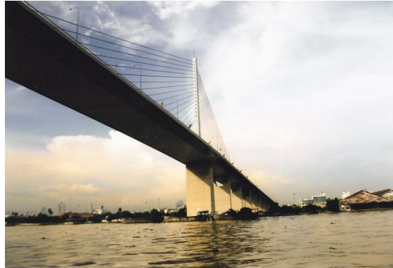
RAMA IX Bridge, Bangkok, Thailand (Photo by Katrin Janberg, www.structurae.net )
