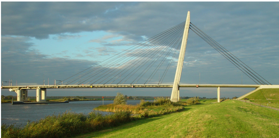
Fig. 65: Cable-stayed “Eiland Bridge” nearby Kampen, The Netherlands, equipped with one MR damper of Maurer Söhne for long-term field tests and damping measurements.
