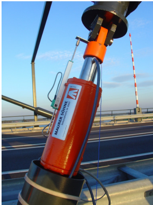
Fig. 83: Displacement sensor and MR damper on the “Eiland Bridge” nearby Kampen, The Netherlands.
