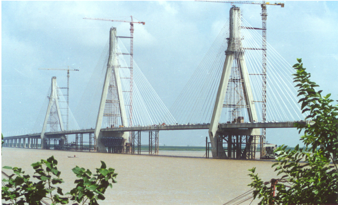
Fig. 64: Cable-stayed “Dongting Lake Bridge” in China, equipped with MR dampers of LORD Corporation.
