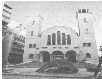
Photo 1.9 Saint Constantine's church in Thessaloniki. Front view of the church; the left hand side steeple fell down after the main shock ( PGA \sim 0.19g ).
