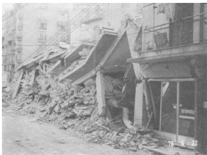
Photo 1.8 Apartment building in Ippodromiou Sq, Thessaloniki. View taken from Nikiforou Foka Str, 30 hours after the collapse.
