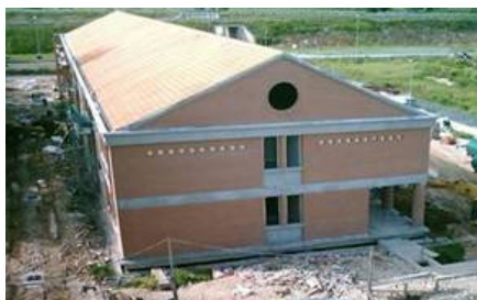
Fig. 15. The isolated fire station (52 HDRBs and 5 SDs), which was recently completed at the Civil Defense Center at Foligno.
