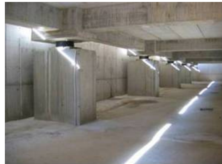
Fig. 16. The new seismically isolated wing of Gervasutta Hospital at Udine, during construction (2005) and view of some of its 52 HDRBs.
