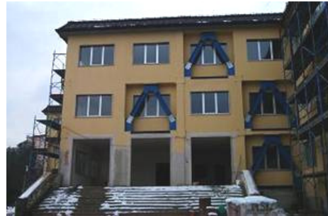
Fig. 13. “Giacomo Leopardi” school at Potenza after its retrofit by means of steel bracings provided with EPDs, similar to the “La Vista” and “Domiziano Viola” schools.
