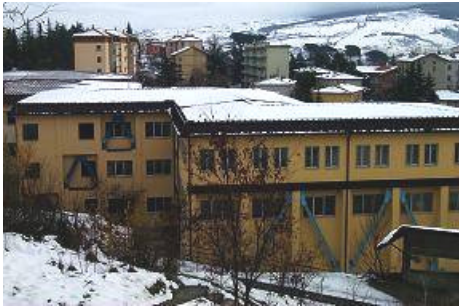
Fig. 13. “Giacomo Leopardi” school at Potenza after its retrofit by means of steel bracings provided with EPDs, similar to the “La Vista” and “Domiziano Viola” schools.
