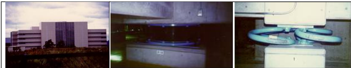
Fig. 1. Ministry of Post and Telecommunications at Sanda City, which withstood the 1994 Great Hanshin-Awaji earthquake without any damage, and details of a RB and an EPD of its SI system.
