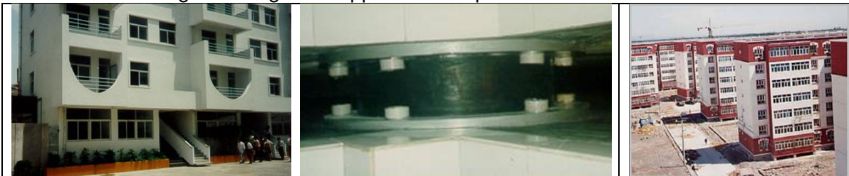
Fig. 5. Dwelling building at Shantou and one of its HDRBs (first Chinese application of modern SVPC systems in 1991), which withstood a significant earthquake without any damage in 1994 (left and center); complex of 60 new masonry dwelling buildings isolated with HDRBs in Western China in 1996 (right).
