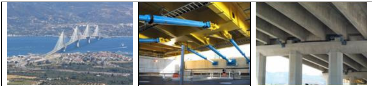
Fig. 29. View of the Rion-Antirion bridge in Greece (12 km long), which has been protected by SVPC devices manufactured in Italy (left); some of the 20 Italian transversal VDs installed in the main bridge (force = 3500 kN, displacement = \pm 1750 \div 2600 mm) (center); some of the 168 Italian transversal and longitudinal VDs in the two approaches (force = 300 \div 2400 kN, displacement = \pm 250 \div \pm 420 mm) (right).
