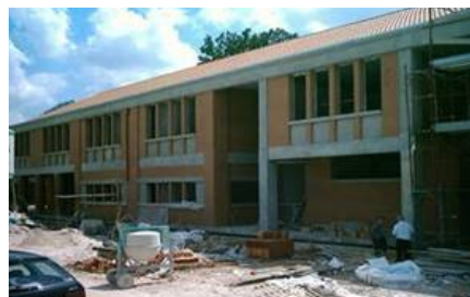
Fig. 15. The isolated fire station (52 HDRBs and 5 SDs), which was recently completed at the Civil Defense Center at Foligno.
