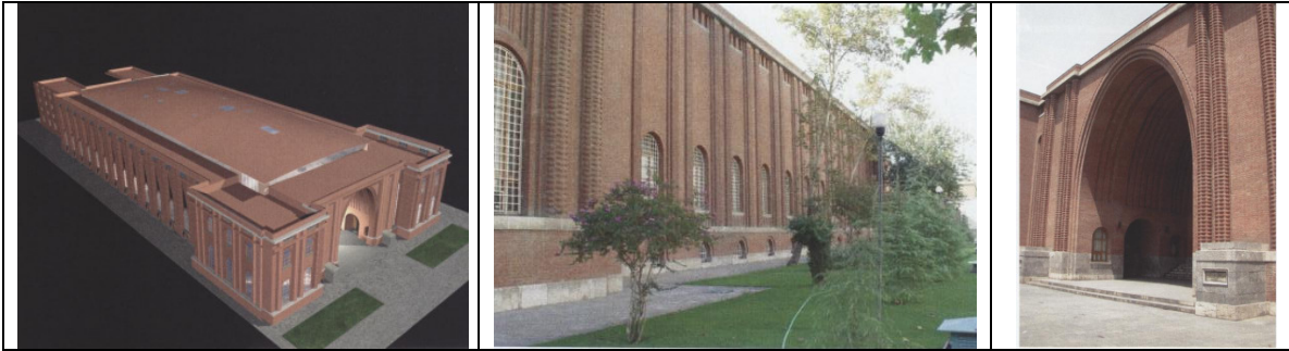
Fig. 33. Sketch and views of the Iran Bastan Museum at Tehran, for which a retrofit design with SI has been developed by a team of Italian designers taking advantage of GLIS and ASS/Si collaborations.
