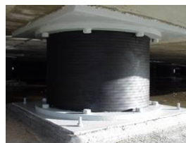
Fig. 27. 140,000 m 3 capacities LNG tank at the Aliaga-Izmir terminal of Egegaz (Turkey) protected by 112 LRBs on the borders and 221 LDRBs internally; view of the isolators during installation and of an installed device.
