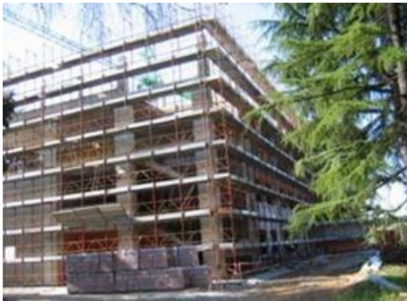
Fig. 16. The new seismically isolated wing of Gervasutta Hospital at Udine, during construction (2005) and view of some of its 52 HDRBs.
