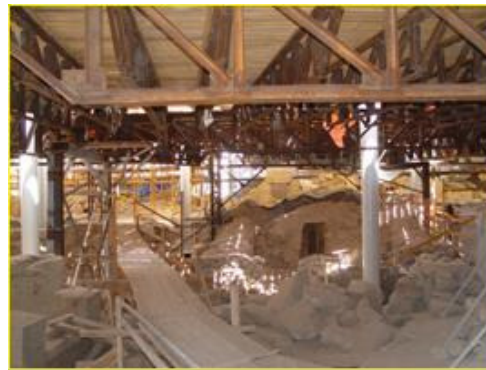
Fig. 31. Reticular ceiling (11,800 m 2 ) of Akrotiri archaeological excavations in the Greek Santorini island, isolated with 92 LRBs and 2 SDs manufactured in Italy in 2003.
