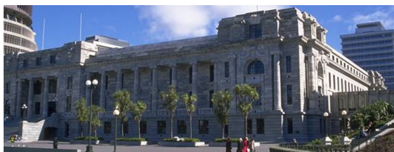
Fig. 25. The New Zealand Parliament at Wellington built in 1921 and seismically retrofitted with LRBs in 1992-93.
