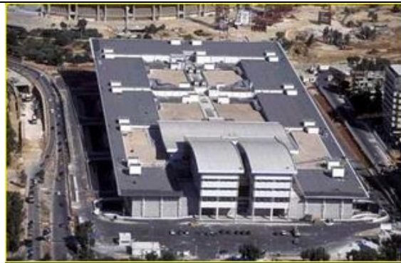
Fig. 30. International Broadcasting Center at Athens (90,000 m 2 total floor area), isolated with 292 HDRBs manufactured in Italy in 2003.
