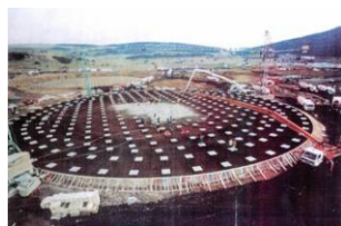
Fig. 27. 140,000 m 3 capacities LNG tank at the Aliaga-Izmir terminal of Egegaz (Turkey) protected by 112 LRBs on the borders and 221 LDRBs internally; view of the isolators during installation and of an installed device.
