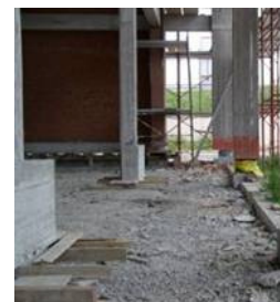
Fig. 15. The isolated fire station (52 HDRBs and 5 SDs), which was recently completed at the Civil Defense Center at Foligno.
