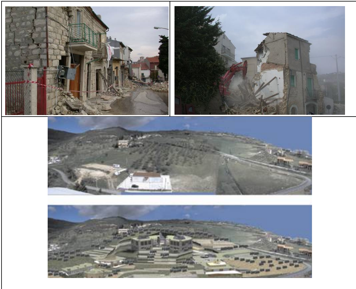
Fig. 12. Views of San Giuliano di Puglia before the 2002 Molise earthquake, as damaged by this earthquake and during and after the demolitions of the debris of the collapsed school and other buildings; view of the site for the erection of the new school (which will be seismically isolated by means of 61 HDRBs and 13 SDs, based on a design coordinated by ENEA) and sketch of the designed construction.
