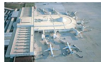
Fig. 28. Retrofit of the Antalya international airport (500 LRBs+SDs).
