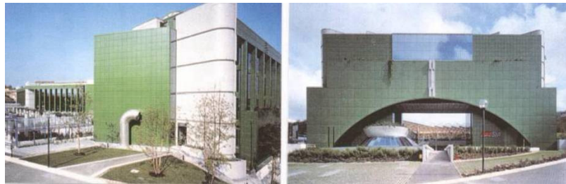
Fig. 11a. Regional Center of Telecom Italia at Ancona, after its completion with 297 HDRBs in 1992 (“rectangular” shape buildings and entrance arch building).
