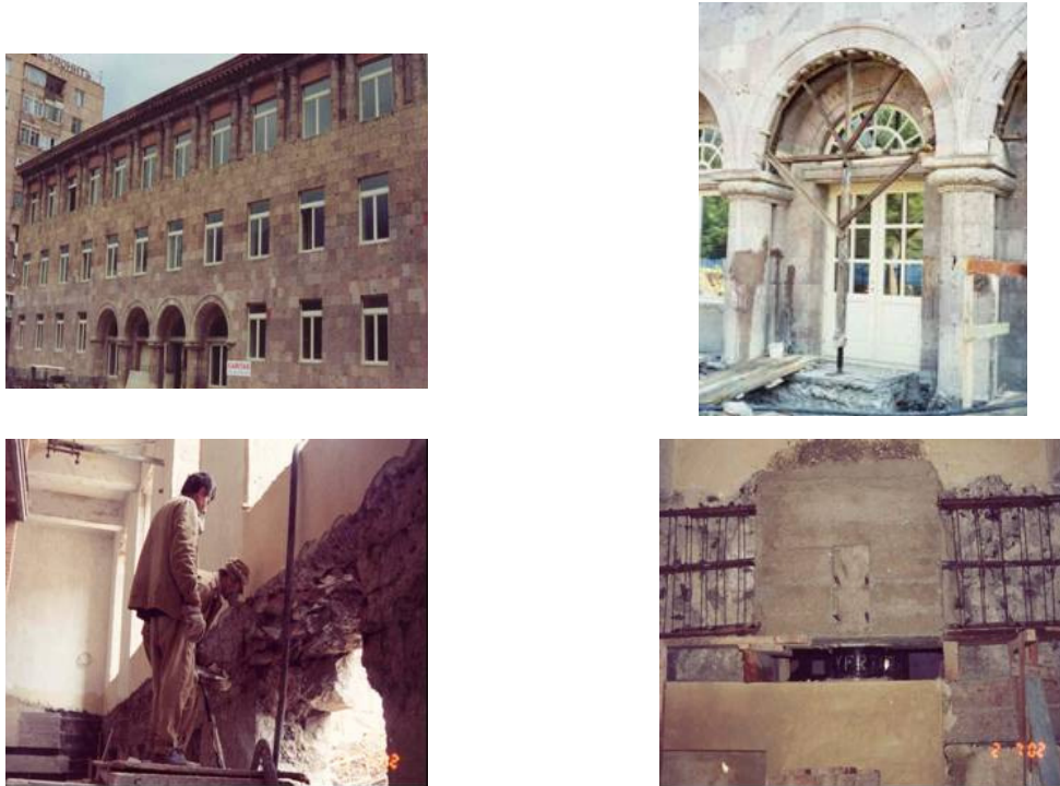
Fig. 24. The masonry school nr. 4 at Vanadzor (Armenia), which was seismically retrofitted with HDRBs in 2002; provisional support of the entrance columns during works; opening of the foundations to insert the new r.c. columns and HDRBs; one HDRB already inserted in the new r.c. column, before the full demolition of the old walls at the beams' positions and casting such beams.
