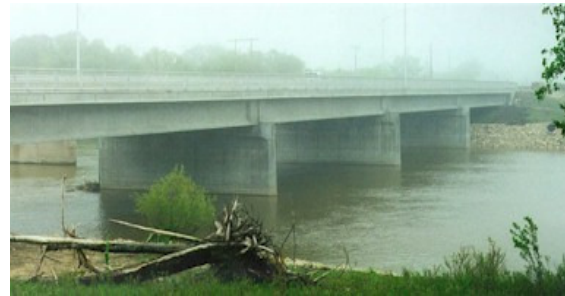
Fig. 7-4. Taylor Bridge in Headingley, Manitoba. Built 1997
