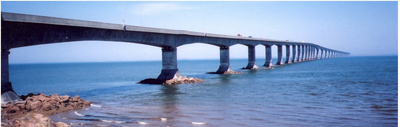
Fig. 7-1. The Confederation Bridge, linking the provinces of New Brunswick and Prince Edward Island, was completed in 1997 and is extensively monitored
