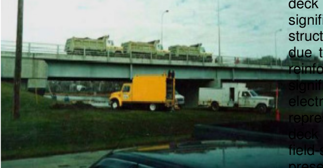
Fig. 7-8. Load testing of the Joffre Bridge with three loaded trucks
