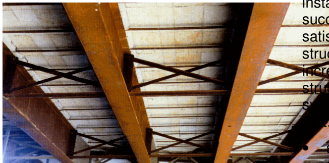
Fig. 7-9. View of the Salmon River Bridge's steel-free deck construction (from below)
