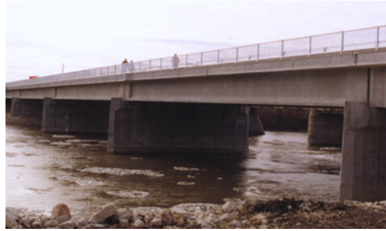
Fig. 1-1. Taylor Bridge, in Headingly, Manitoba, incorporates numerous sensors into its design. In this way, the bridge is capable of sensing loads and deformations and conveying that information to engineers at a remote location. The Taylor Bridge thus exemplifies structural health monitoring, and is an example of one of the world's first "smart" structures
