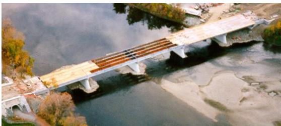
Fig. 7-6. The Joffre Bridge in Sherbrooke, Québec. During reconstruction in 1997
