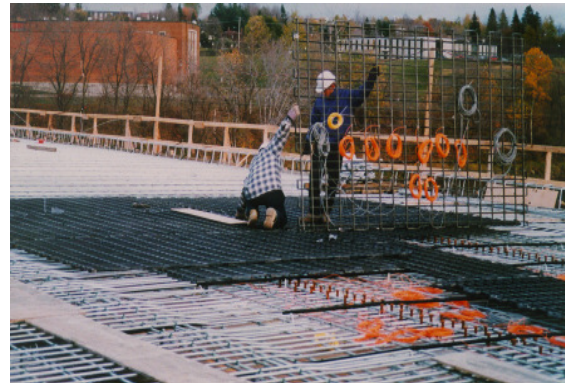
Fig. 7-7. Installation of the instrumented sections of bridge deck reinforcement in the Joffre Bridge
